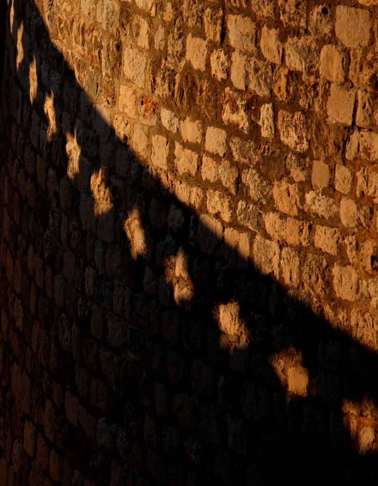
Dubrovnik, wall detail
