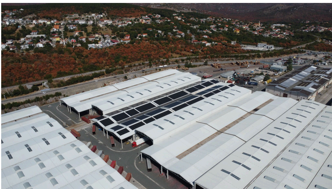
Škrlevo Terminal – a view of the storage infrastructure and solar power plant
