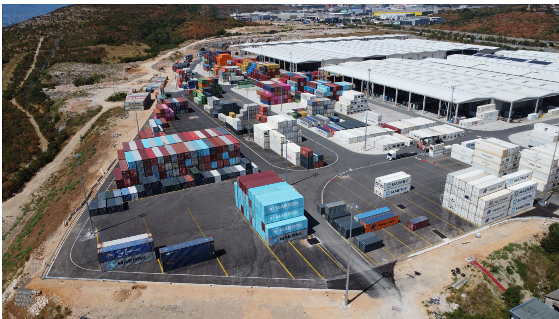
Škrljevo Terminal – container depot and handling areas
