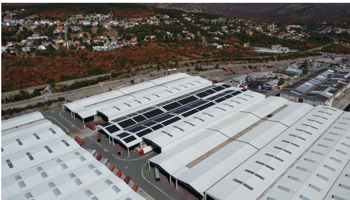
Škrljevo Terminal – a view of the storage infrastructure and solar power plant
