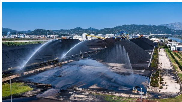
The bulk cargo terminal is equipped with a spraying system that is automatically activated to prevent the release of coal dust.
